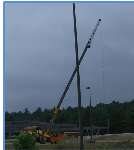
Figure 3: Telescoping Mobile Crane used on site
